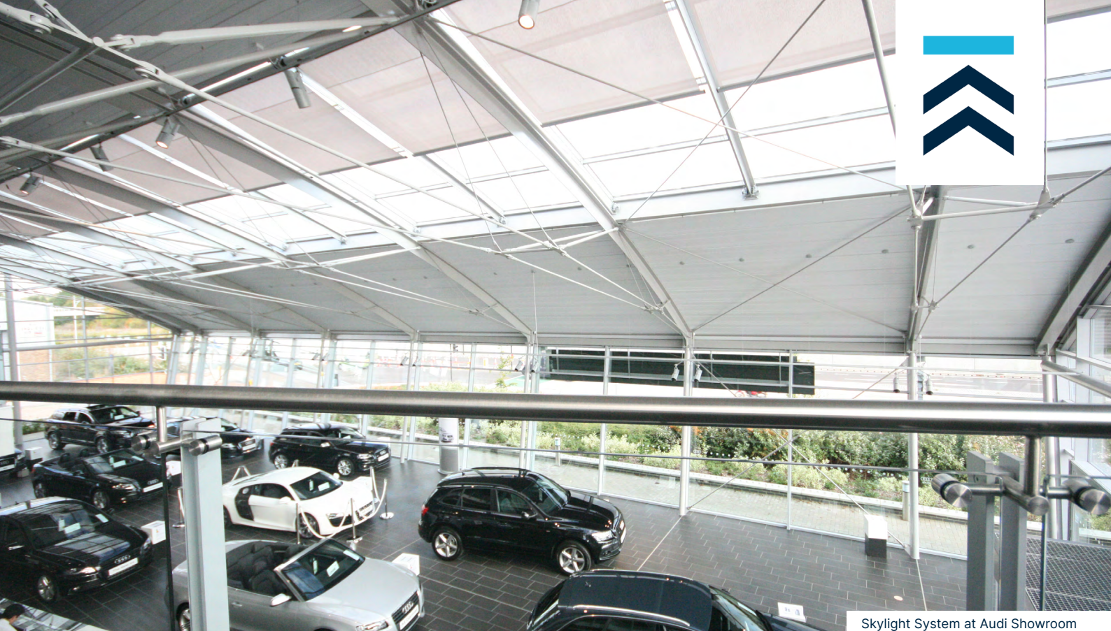
Skylight System at Audi Showroom
